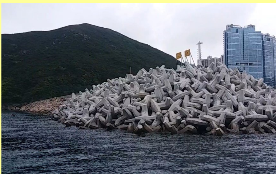
Example: Precast wave breaking units
