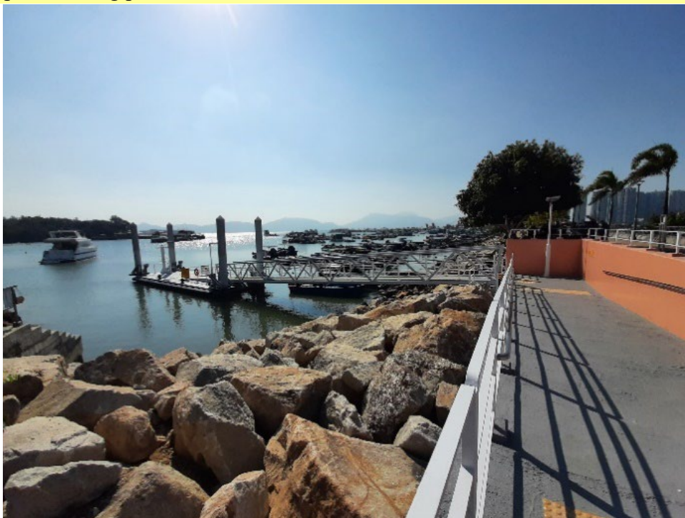
Example: Floating pontoon at Tuen Mun Area 27
