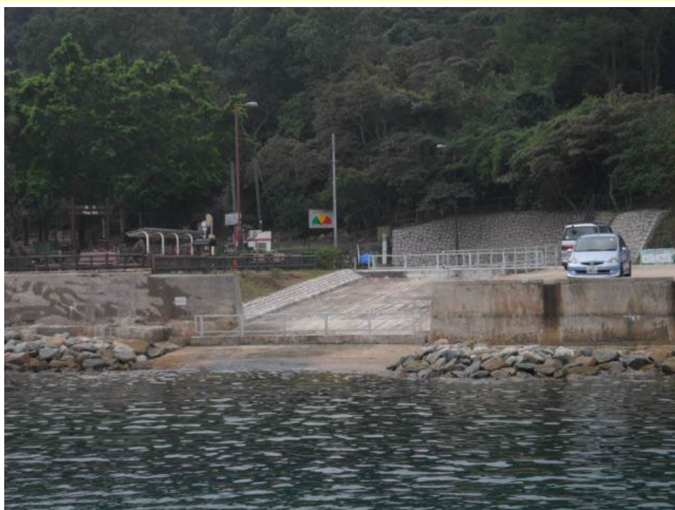
Example: Wong Shek Slipway
